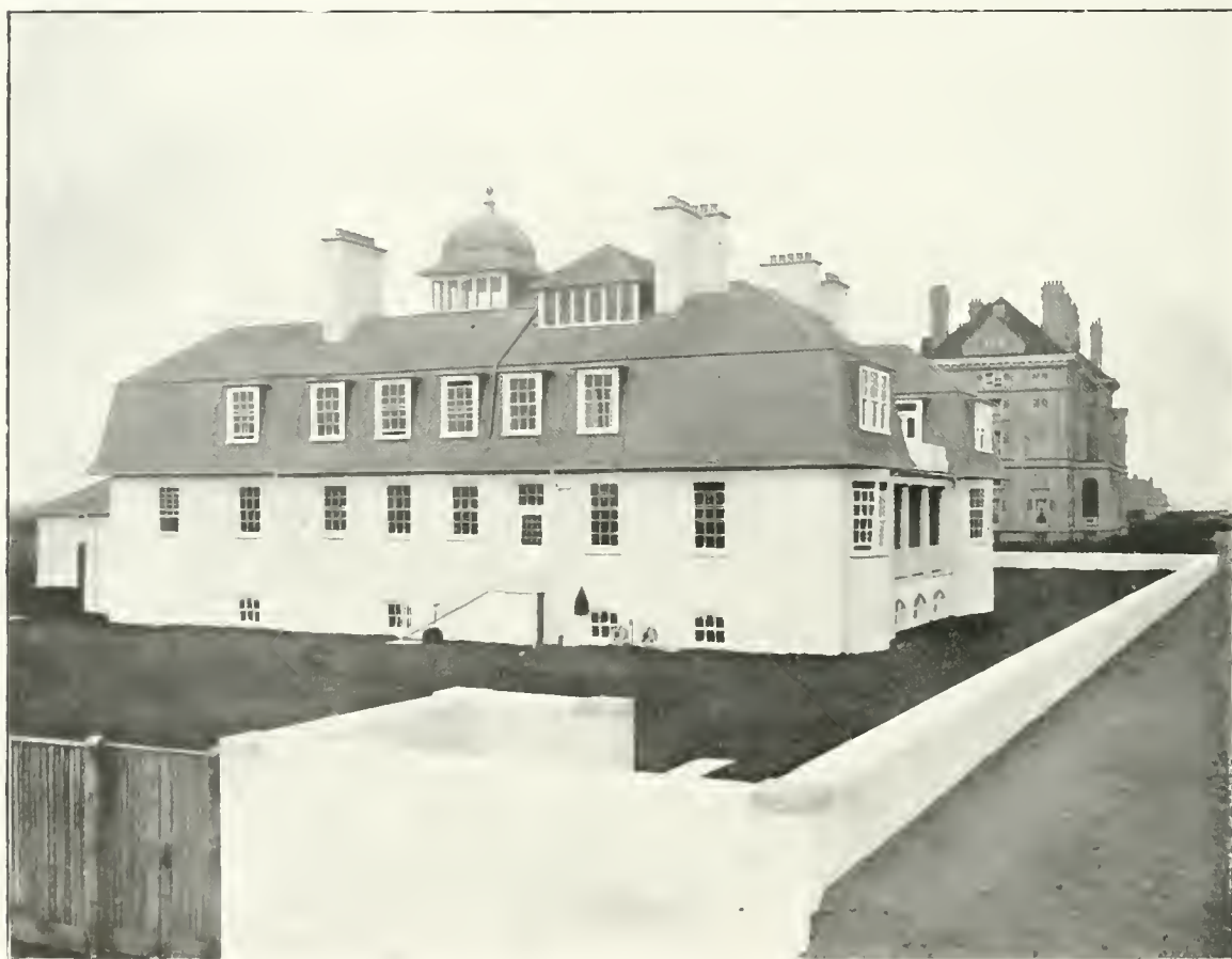
This house is built on the edge of the shore between the Deal and Sandwich Golf Links, and the sea water penetrated within 2 ft. of the footings at high tide.
